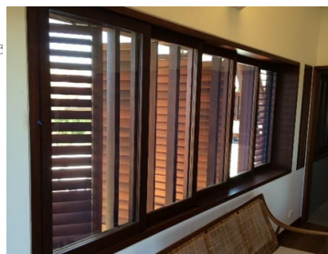
Figure 19b, Timbered louvered windows
