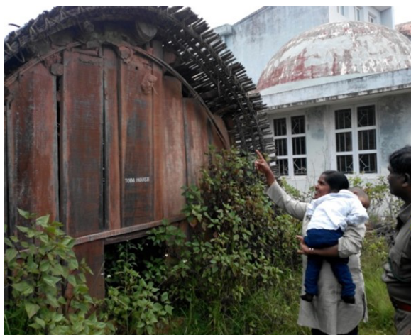
Figure 1: Traditional huts of Toda community. Source: Author
